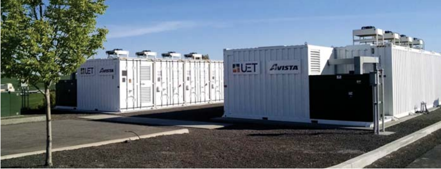
1 MW 4 MWh containerized vanadium flow battery owned by Avista Utilities and manufactured by UniEnergy Technologies
