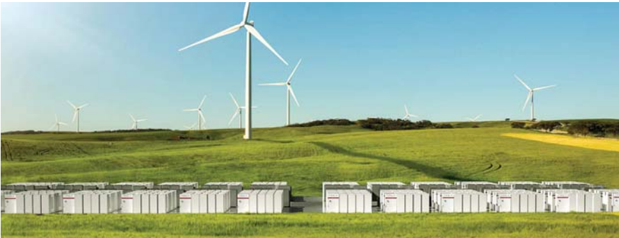
The 129 MWh Powerpack battery, provided by Tesla, integrated into the power grid in South Australia. While far larger than required for the purposes of BSX, this installation illustrates the scalability of Li-ion battery technology. | Image: Tesla
