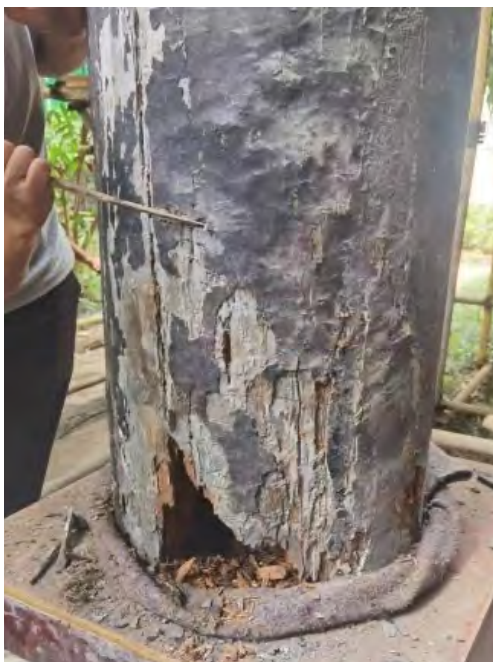
Figure 3.9: Damage due to termite infestation at Chunyang Guan. Photo by Dan Changrong.
