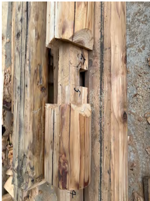
Figure 2.5: Traditional joinery method. Photo by Author.
