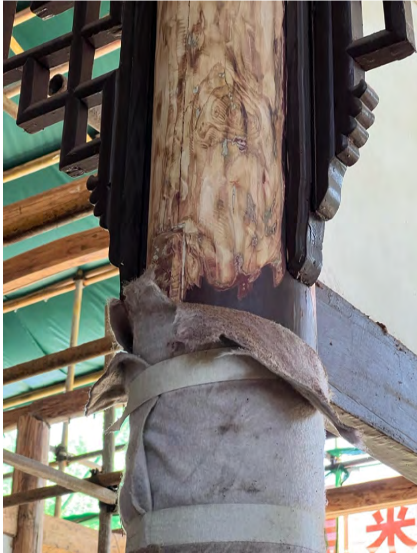
Figure 2.7: Repaired wood component of Chunyang Guan. Photo by Author.
