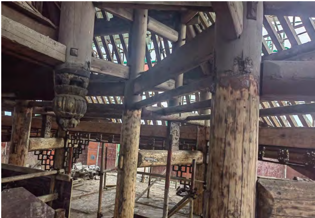
Figure 3.10: Repair of mortise and tenon joints at Chunyang Guan. Photo by Author.
