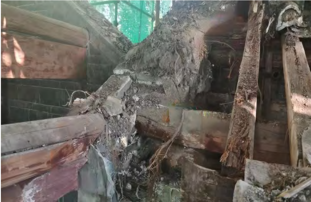
Figure 2.2: Wood decay in Chunyang Guan. Photo by Dan Changrong.
