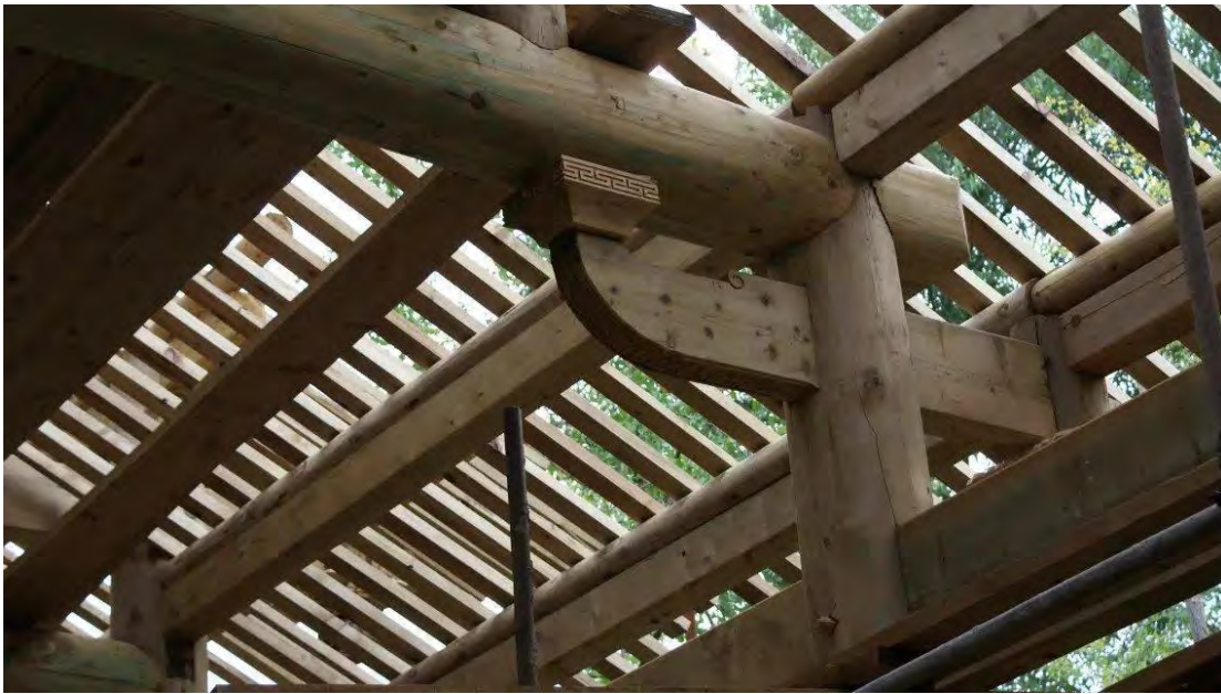
Figure 1.7: Mortise and tenon joints used in ancient wooden temples restoration. Photo by Dan Changrong.
