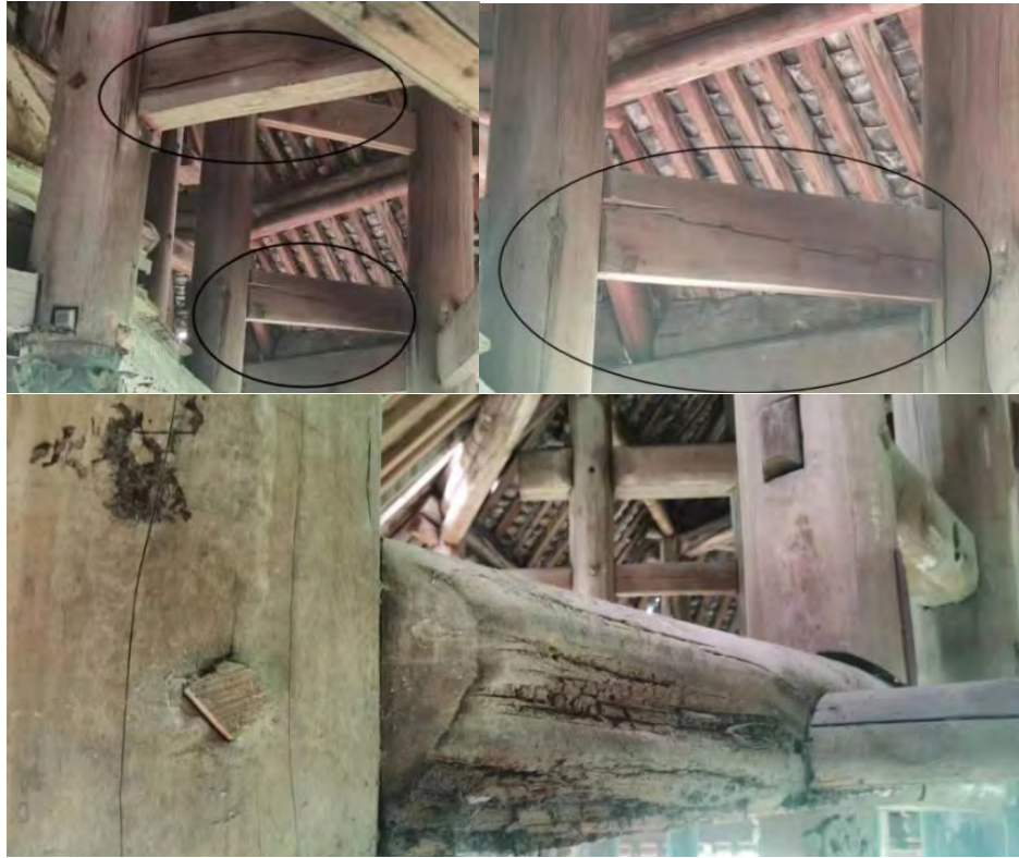
Figure 2.3: Component decay and cracking in Chunyang Guan. Photo by Dan Changrong.
