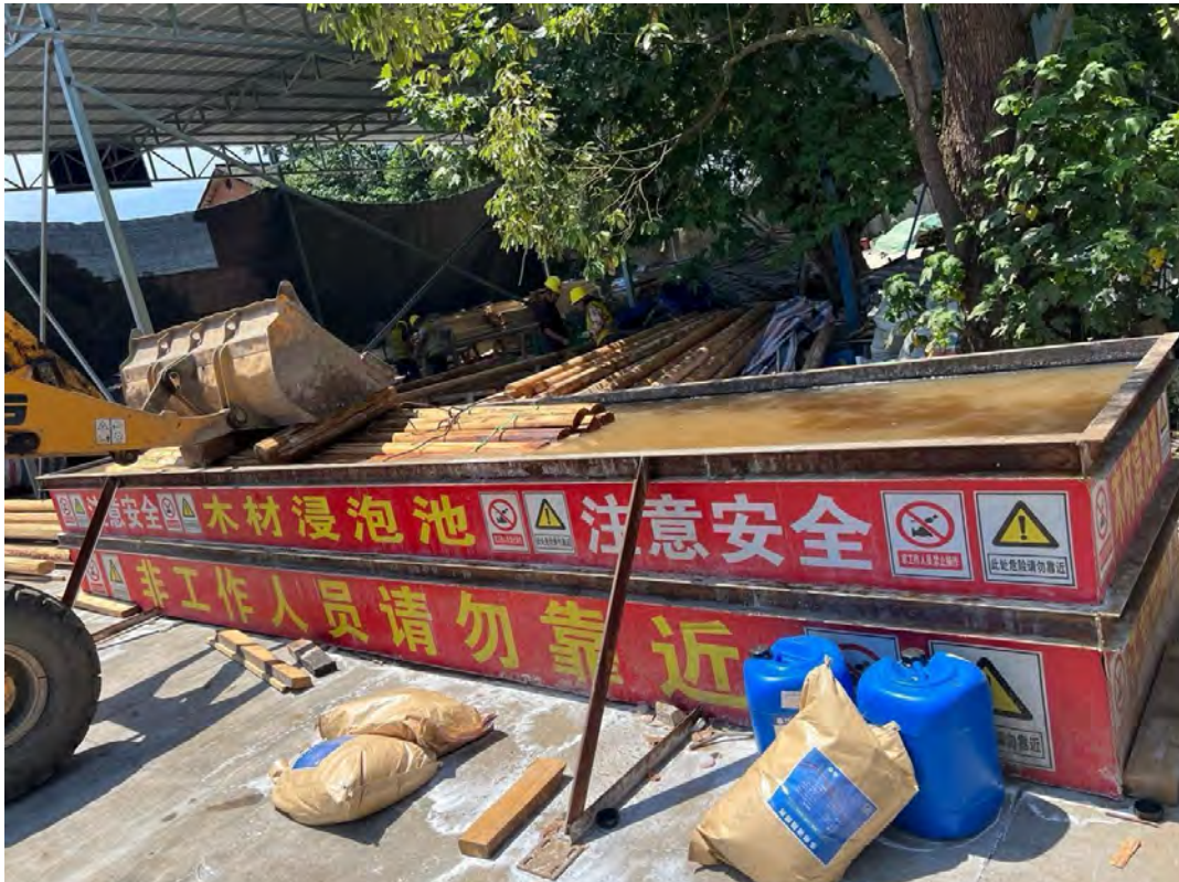
Figure 2.6: Soaking wood in medical solution, such as polyethylene glycol, to prevent cracking and infestation. Photo by Author.
