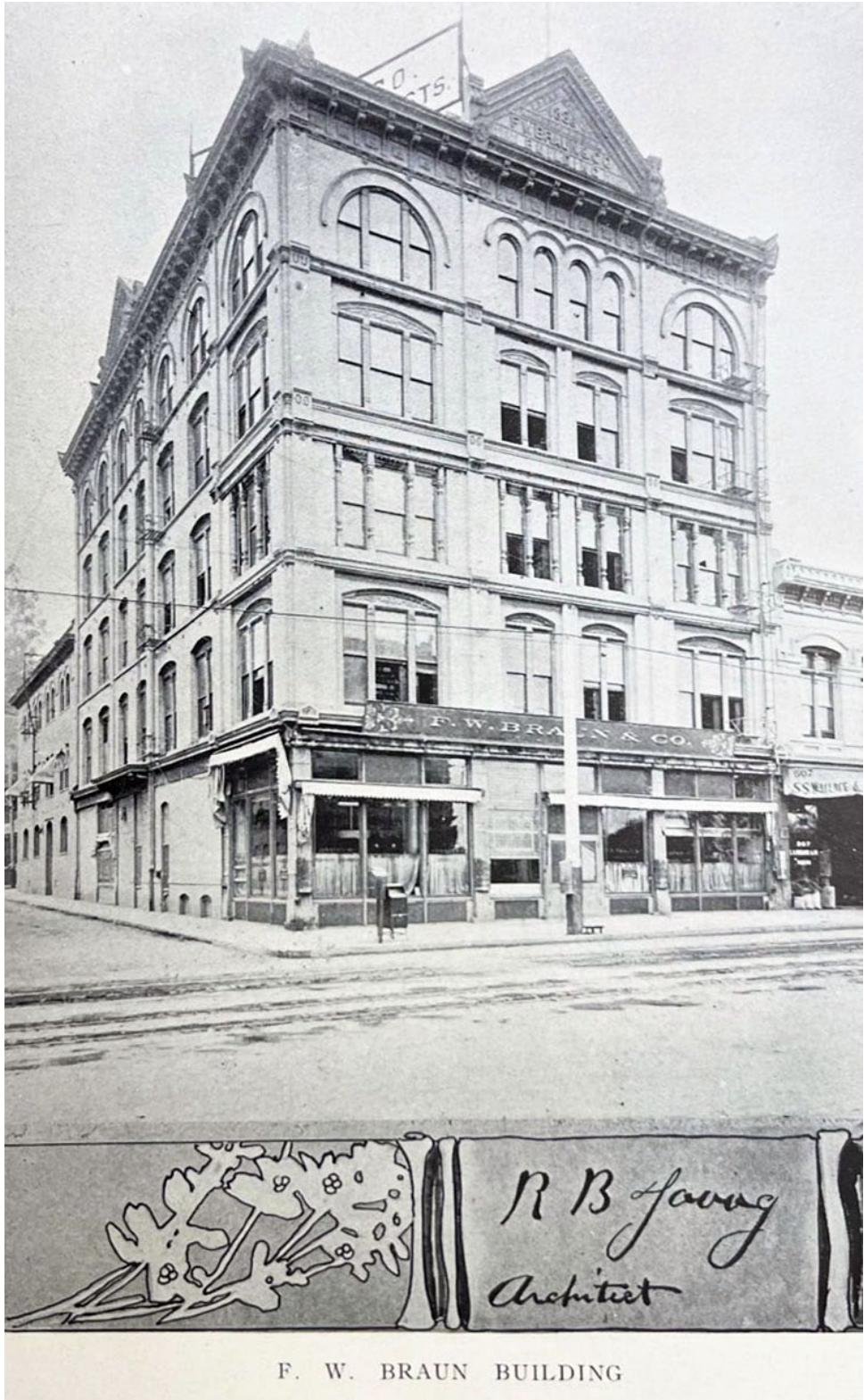
Figure 6.5. F. W. Braun Building.
