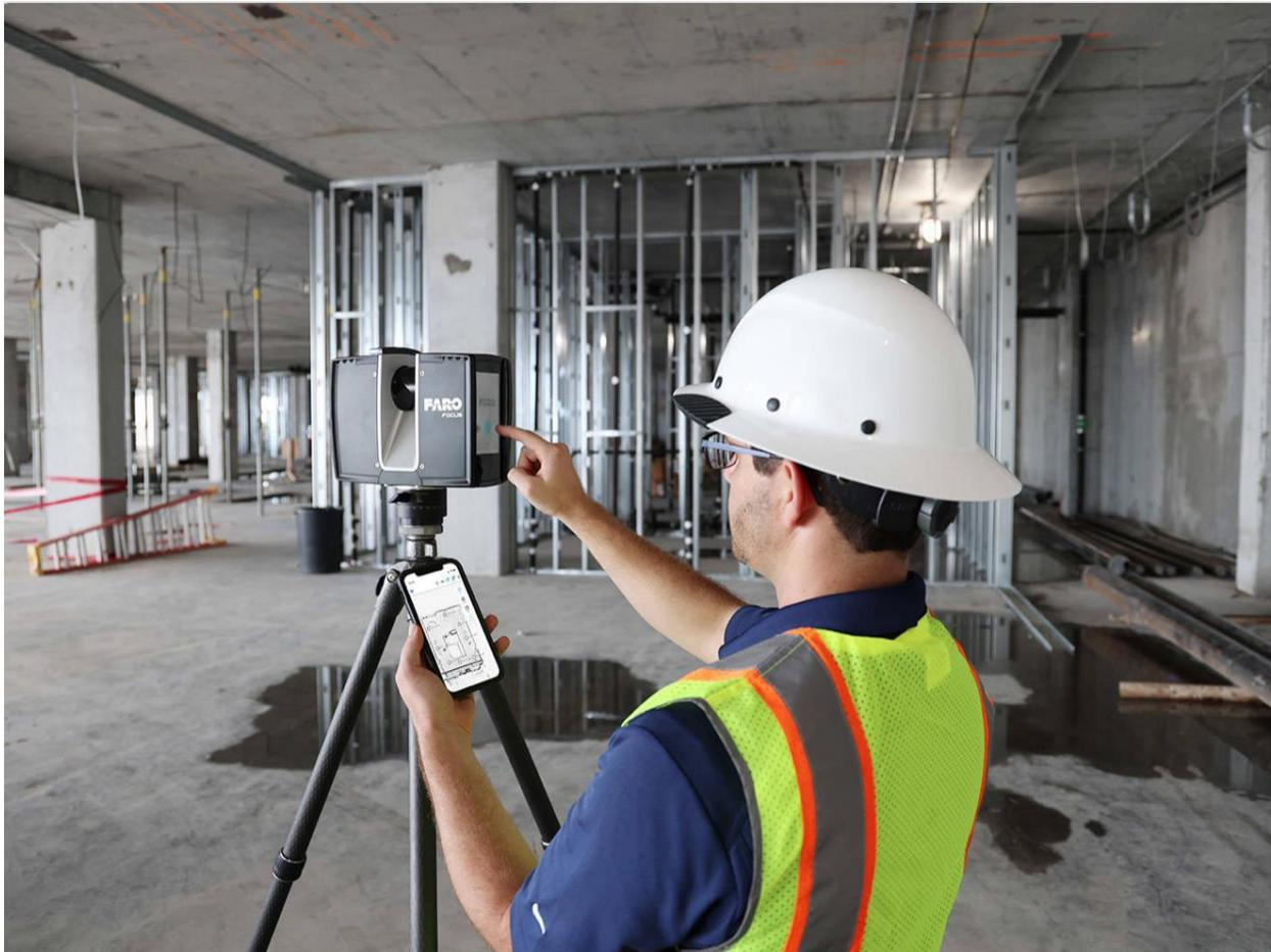
Figure 2-5: Phase Comparison Scanner (Faro, 2022a)
