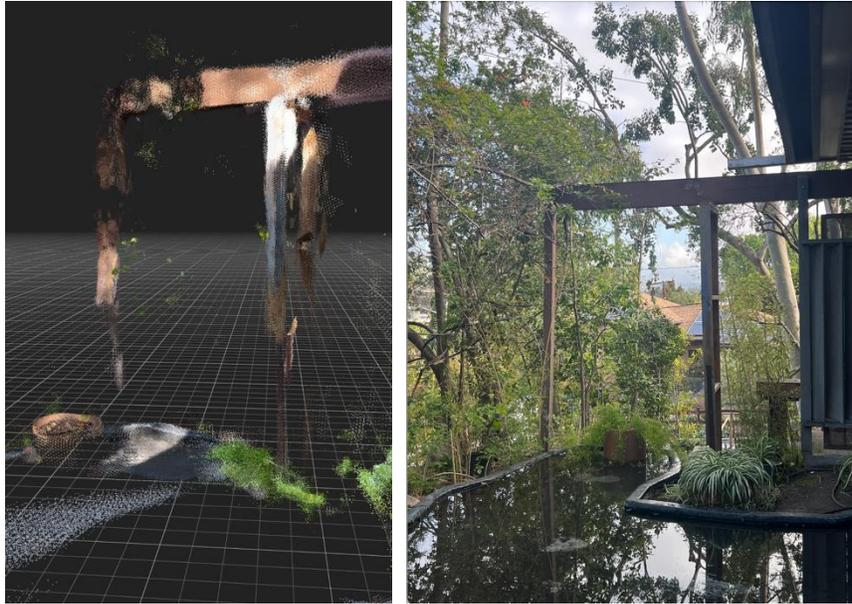
Figure 6-9: “Spider leg” feature detail in iPhone captured point cloud.
