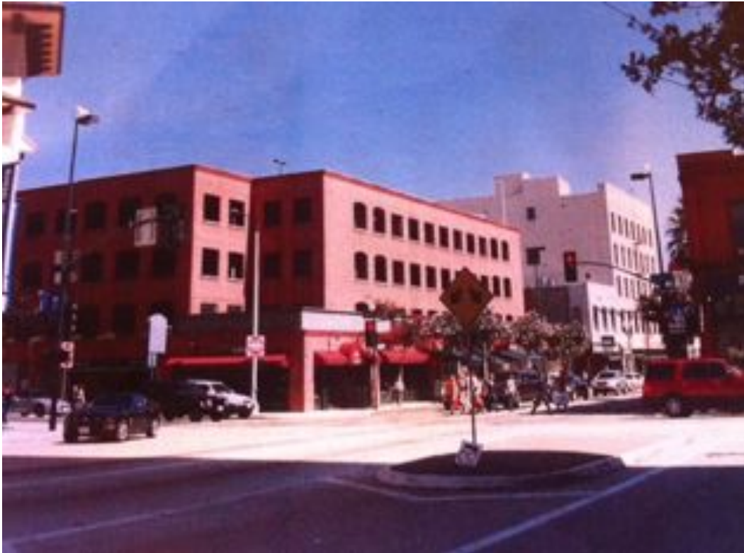
Figure 2.3: Old Town Pasadena Parking Garage. Courtesy of Rood, "Parking Once in Old Pasadena."
