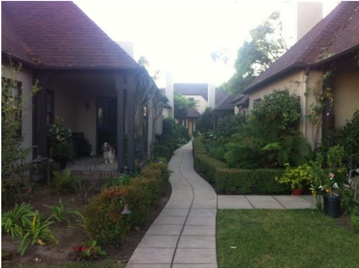
Figure 5.1: Hasket Court by Heritage Housing Partners, Pasadena. Photo by Author.
