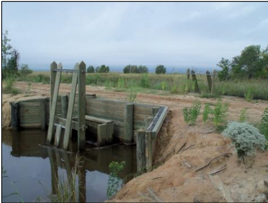
Figure 1.4: Rice Trunk Water Control Structures at Ace Basin National Wildlife Refuge. Image Source: U.S. Fish & Wildlife Service.
