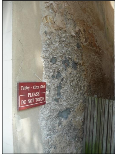
Figure 4.6: Exterior of 715 Bay Street, Beaufort, SC showing exposed tabby construction. Image Source: Cheryl Warren.
