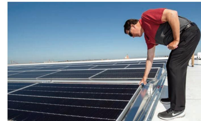
Solar panels will supply as much as 15% of Galen Center's electricity and produce 915,000 kilowatt-hours annually — enough to power 88 houses for a year.
