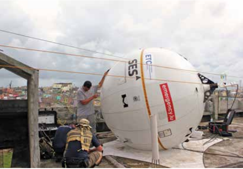
Emergency.lu setting up satellite communications after a disaster.
